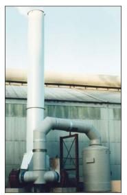
During operation, the gas to be cleaned flows vertically upward into the tray section through the sieve holes or capped risers, which can vary up to 1-inch diameter. Scrubbing liquid is introduced to the top trav where it flows in a horizontal cross flow direction to the gas rising over the tray's surface. The gas velocity through the trav openings. holds the liquid up on the trav and creates a froth layer where violent gas and liquid contact occurs to
