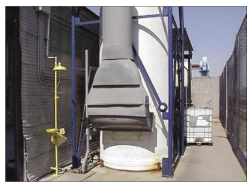
The bottom section of the scrubber shown in with tote container of BIONOxSOLVER.
